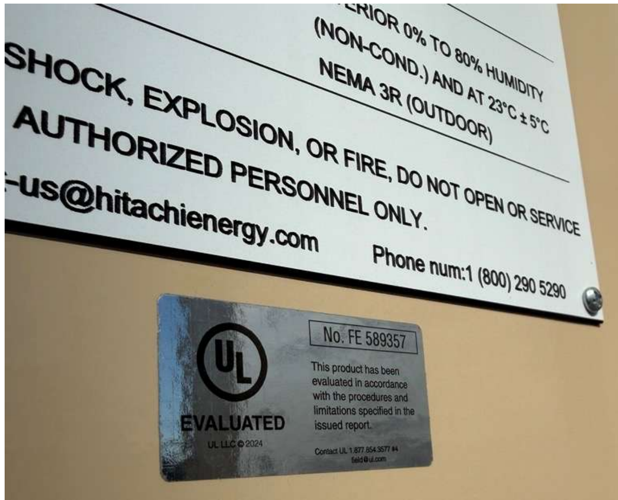
Figure 5. UL Field Evaluation Product Label as observed on the BESS enclosure in the field.
